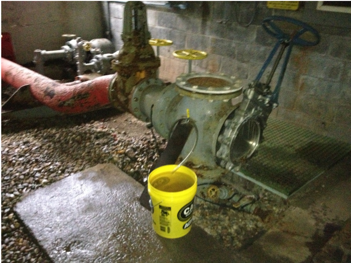
Figure 16. A small valve allows the sampling of water from the pipe carrying water from Laurel Lake to the Housatonic River at the old Eagle Paper Mill in Lee, MA.
