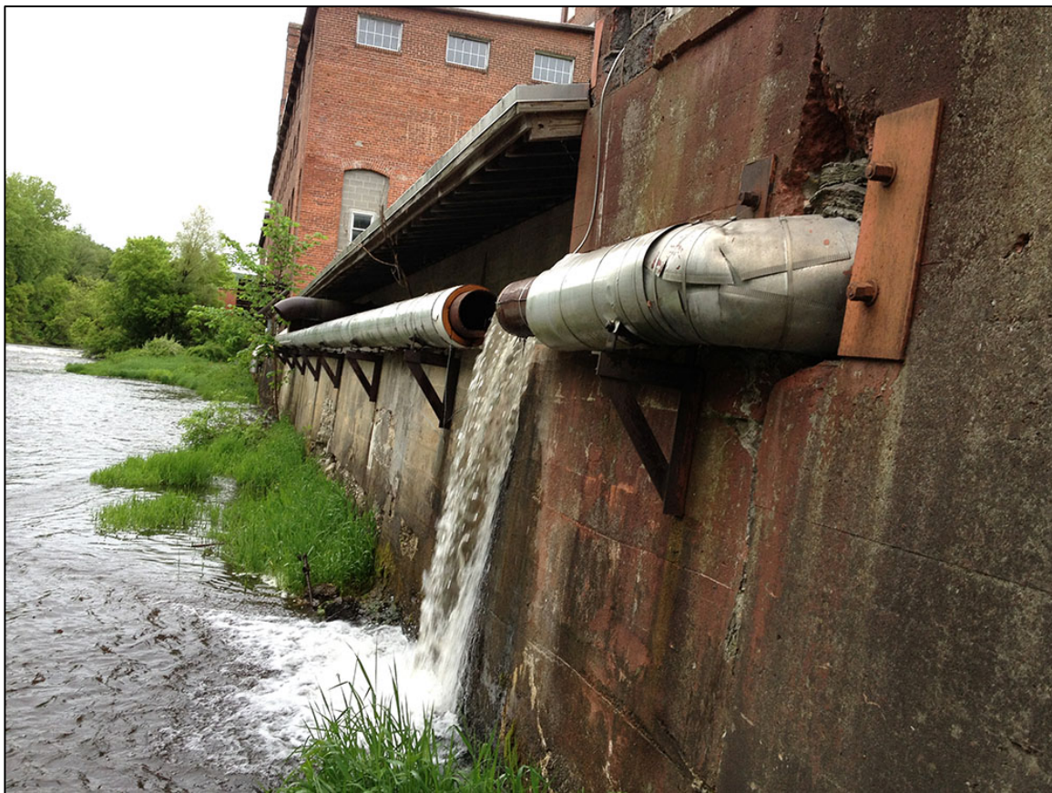
Figure 15. The pipe carrying water from Laurel Lake empties into the Housatonic River at the old Eagle Paper Mill in Lee, MA.
